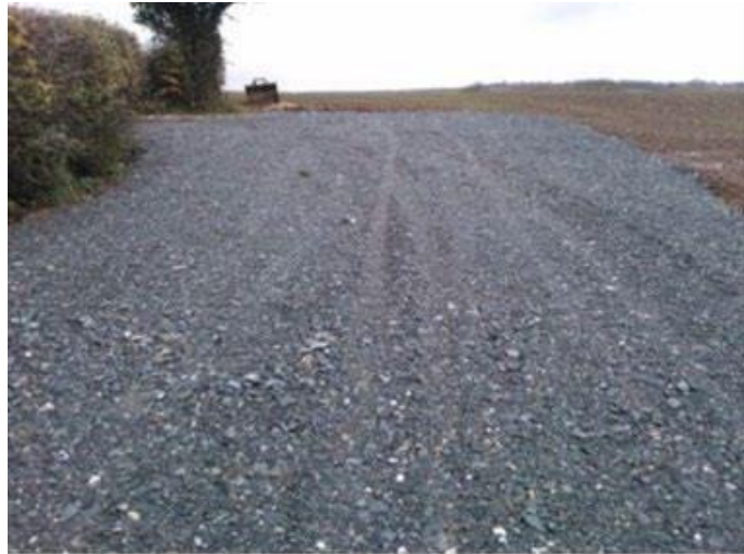
Figure 4 – Example Access track
