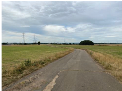
Photograph 7: Hardstanding roads, view from north to south within centre of site
