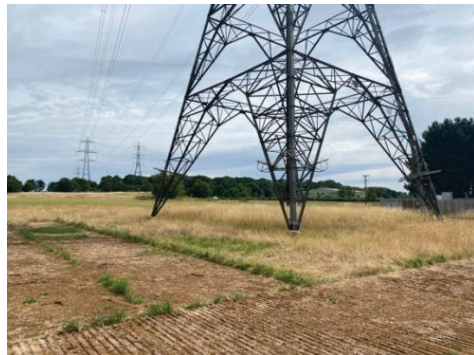
Photograph 9: Bare ground beneath pylon
